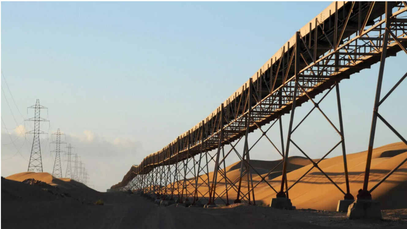
PHOSPHATE CONVEYOR, BOUCRAA, WESTERN SAHARA (PHOTO VIA WWW.MEM.GOV.MA )
